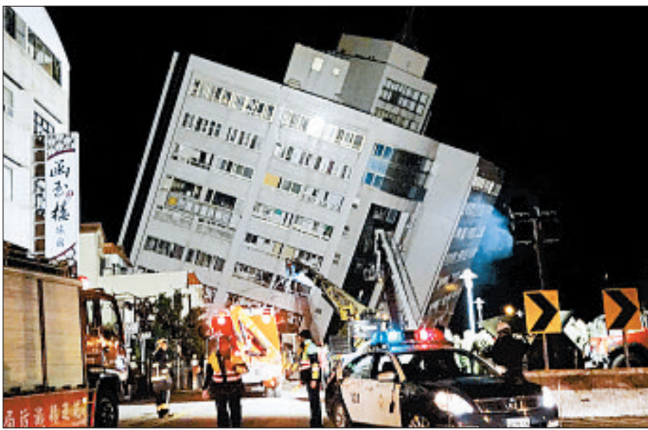
Deadly quake in Taiwan: Rescue crews search a building that partially collapsed Wednesday in Taiwan after a 6.4 magnitude quake. Officials said four people in Hualien County were killed and more than 200 injured. More than 140 were unaccounted for.
