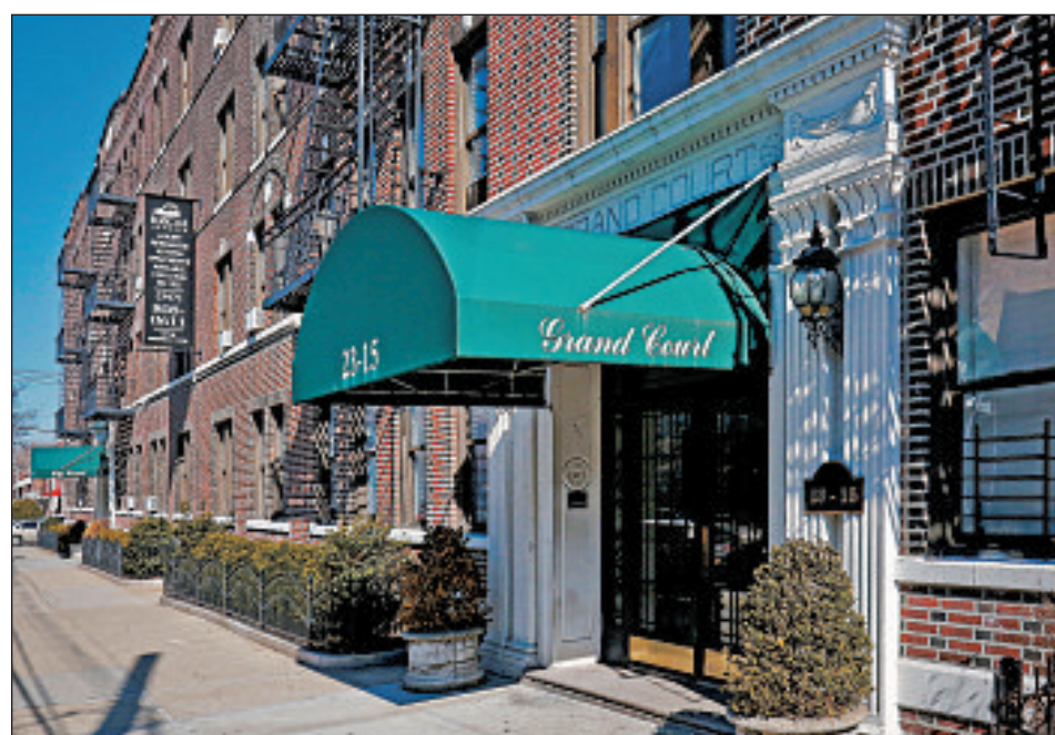
Kushner Cos. filed construction permits on three buildings in Queens, N.Y., including this one, declaring it had zero rent-regulated tenants.
