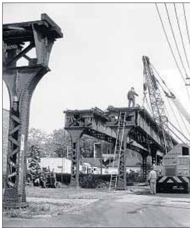
Workers tear down the Humboldt Park “L” branch, which ran from near the Damen stop west to Lawndale Avenue.
