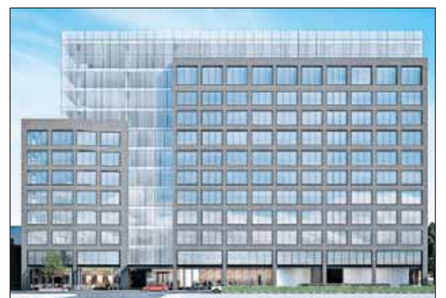
The building would be airtight and heavily insulated to trap air-conditioned or heated air for longer periods of time.
