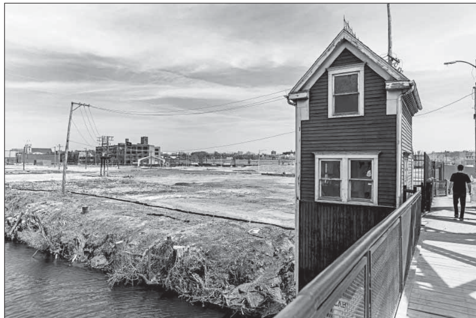
The former A. Finkl & Sons steel plant site, viewed from the Cortland Street bridge.
