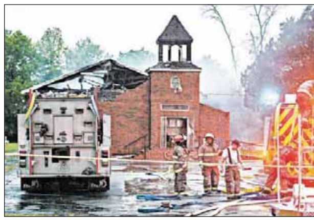
LESLIE WESTBROOK/THE ADVOCATE Firefighters and fire investigators respond to a fire April 4 at Mount Pleasant Baptist Church in Opelousas, La.
