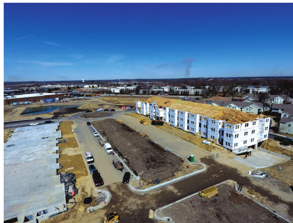
Construction continues on Prairie Centre in St. Charles with the first apartment building under roof and another underway.
