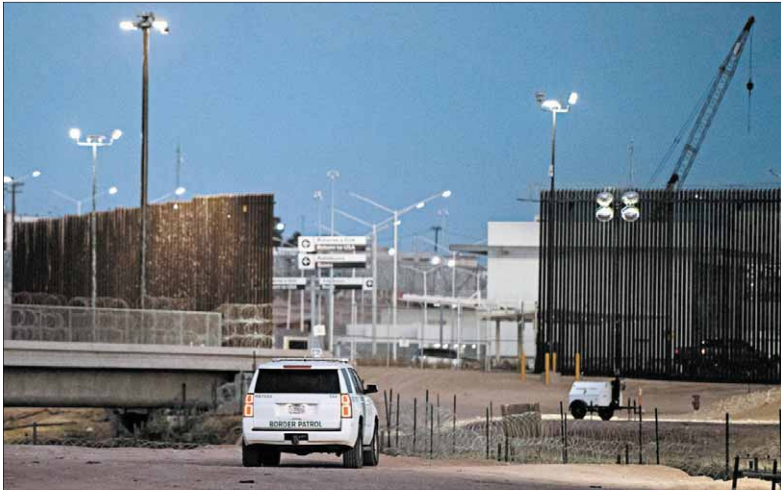
CAROLYN VAN HOUTEN/WASHINGTON POST In Calexico, California, a section of border fence, right, was painted black to absorb heat, something President Trump hopes will deter climbers.
