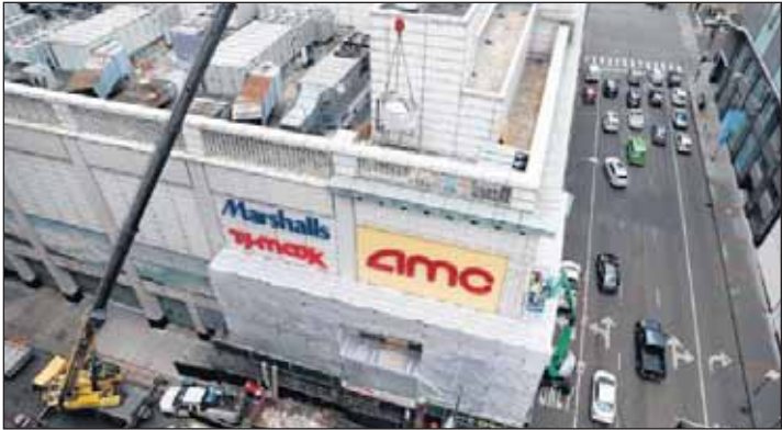
ANTONIO PEREZ/CHICAGO TRIBUNE With the help of a crane, riggers guide brewery equipment down and into the soon to be opened Crushed by Giants brewery Monday in downtown Chicago.
