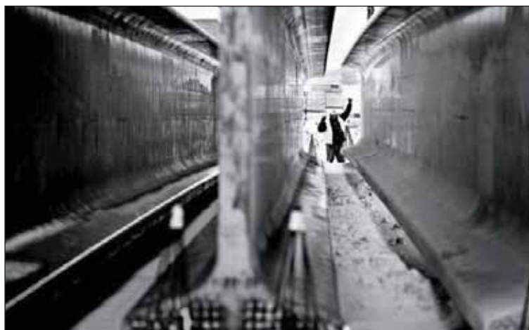
Juan Pedroza guides the lowering of an 187-foot precast prestressed concrete beam in the shipping yard at County Materials Corp.
