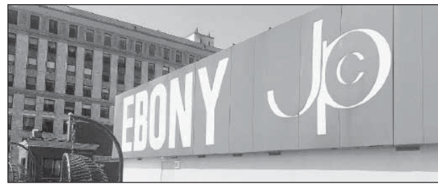
The former Johnson Publishing building is pictured at 820 S. Michigan Ave. in Chicago.
